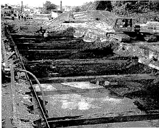
Photo 2. Excavation with secondary sheet piling shoring.
